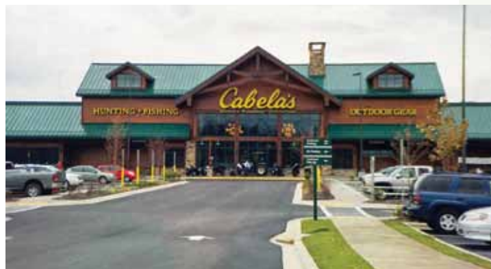
Anchored by the first Cabela's in the state, The Falls is a 140-acre development with over 1,000,000 square feet of retail space. With $22 million in road improvements and over two million projected shoppers annually, the Falls is one of the top retail tourism developments in the state.
